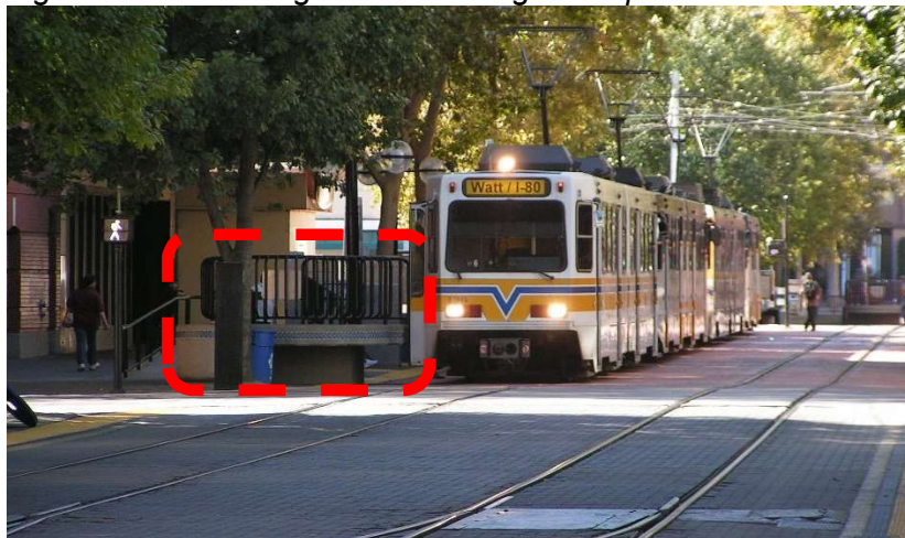
Figure 28: SacRT Light Rail Mini-High Ramp
