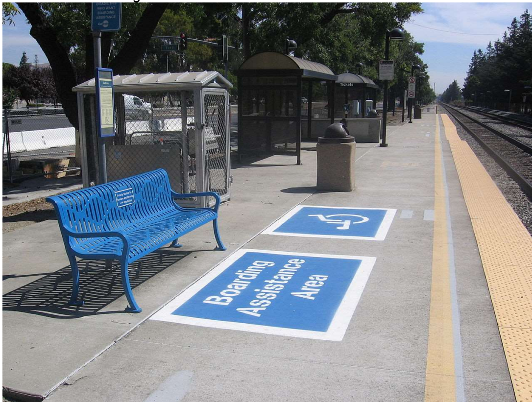
Figure 34: Platform Markings for ADA Access
